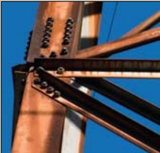
towers that are closest to transitioning from one phase of corrosion to the next. This saves several thousand dollars in repair costs per tower and also helps owners identify which towers should be repaired first and which ones can be fixed at a later date.
