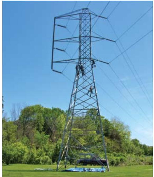
Workers paint an energized 138-kV double-circuit angle with a special coating from PPG North America.
