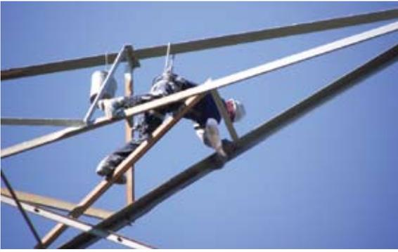
After linemen inspect the towers, painters then use mittens to paint a steel arm on a transmission tower.
